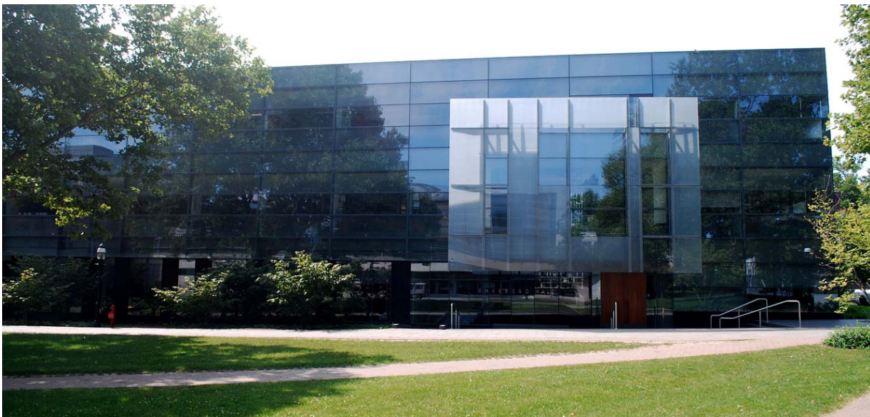
Figure 6: Daytime Image of Façade at Main Approach
